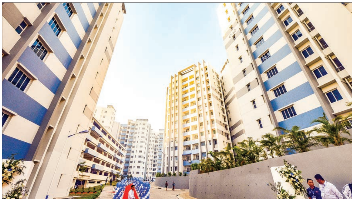
Photo shows the two housings for university teachers in Hline Township, Yangon, yesterday. PHOTO: MNA
