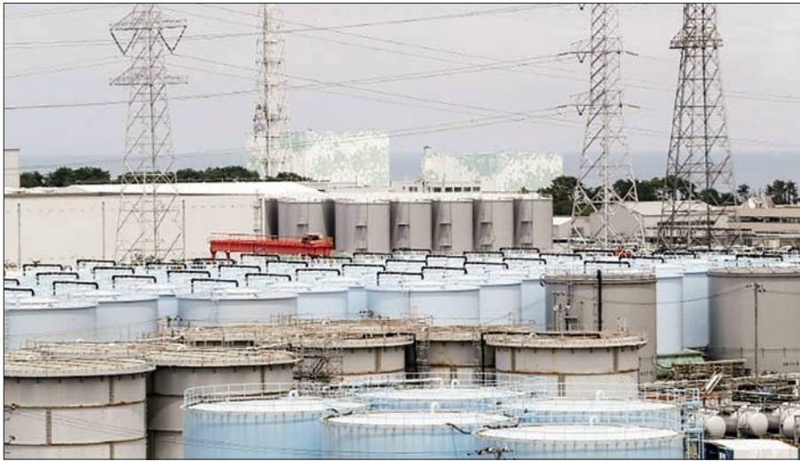
Storage tanks holding radioactive water at Japan's crippled Fukushima power plant. PHOTO: AFP
