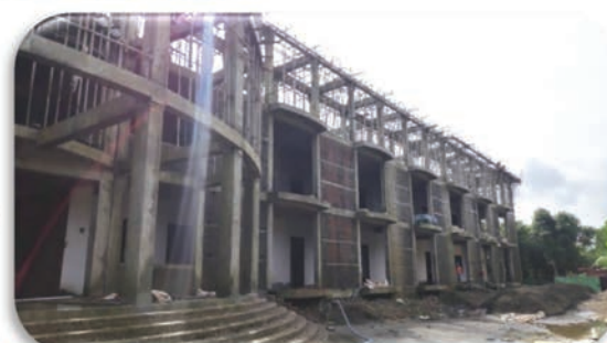
Construction of 3-Storey Main Building at Technology University (Sittwe)
