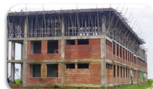
Construction of 3-Storey Classroom Building at Sittwe University
