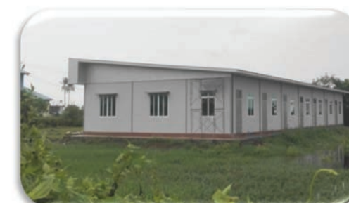
Construction of 7-Unit Canteen at Sittwe University
