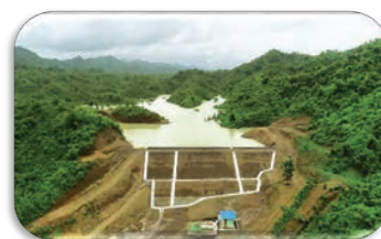
Construction of Yotayoke Hillside Dam in Ponnakyun Township
