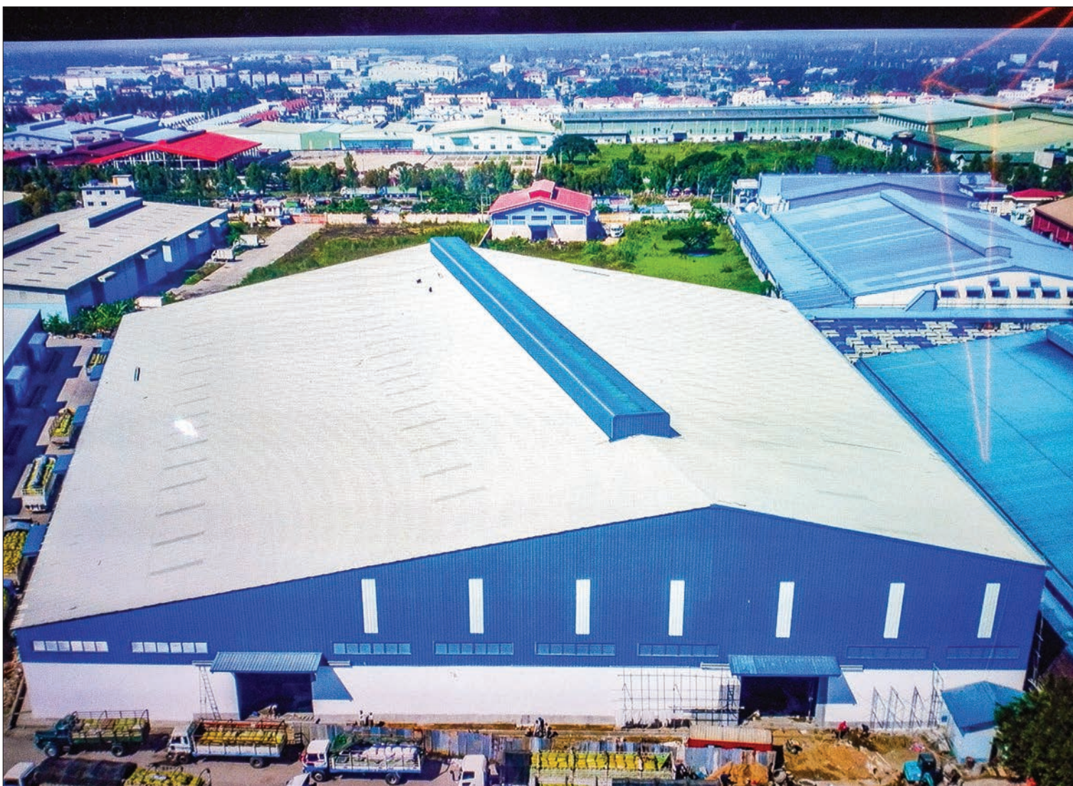
A bird's-eye view of PEB Steel Myanmar's steel plant. PHOTO: MYINT MAUNG SOE
