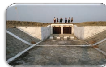
Construction of 2 Concrete Sluice Gates in Minbya Township
