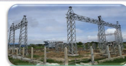
Construction of Hsat Yoe Kya Electric Power Sub-Station
