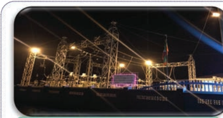
Construction of Zinchaung-Saneh Electric Power Sub-Station
