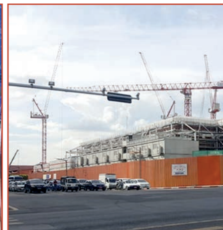
Yoma Central project site PHOTO: YE HTUT TIN (NLM)
