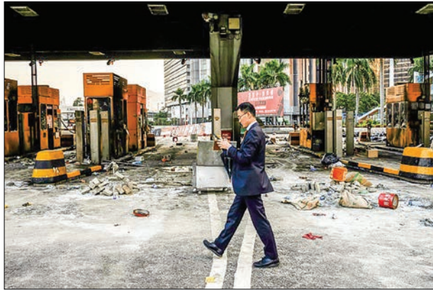
The Cross Harbour Tunnel has been blocked since Tuesday. PHOTO: AFP
