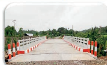
Construction of Let Pan Su Bridge on Thandwe-Kinmaw Road
