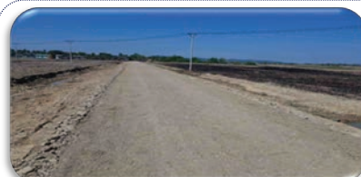
Construction of rural connectivity road in A-wa Village in Minbyar Township
