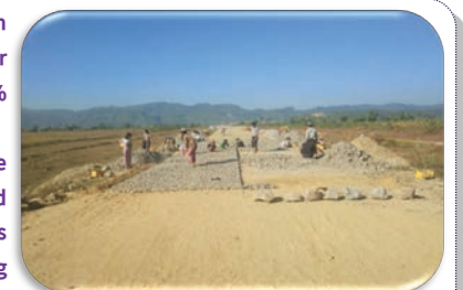
Construction of Kyauk Pandu-Inndin-Zedi Pyin Road
