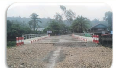
Construction of Ram Thit Kye Bridge on Peinne Taung-Ramree Road
