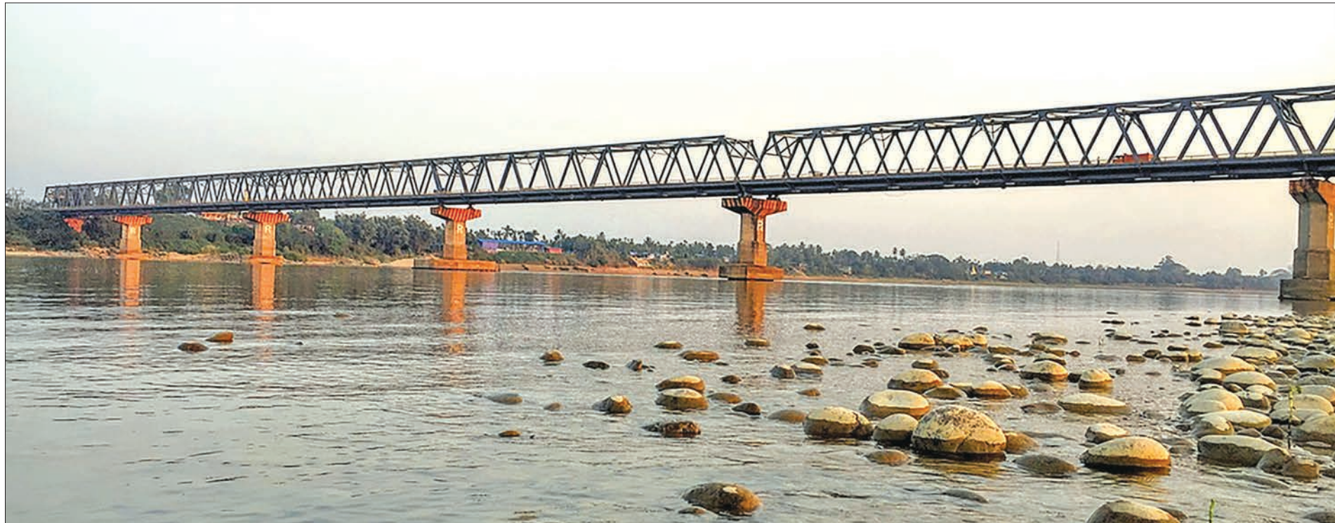
Balaminhthin Bridge No.1 in Myitkyina, Kachin State. PHOTO: HTEIN NAN NAW
