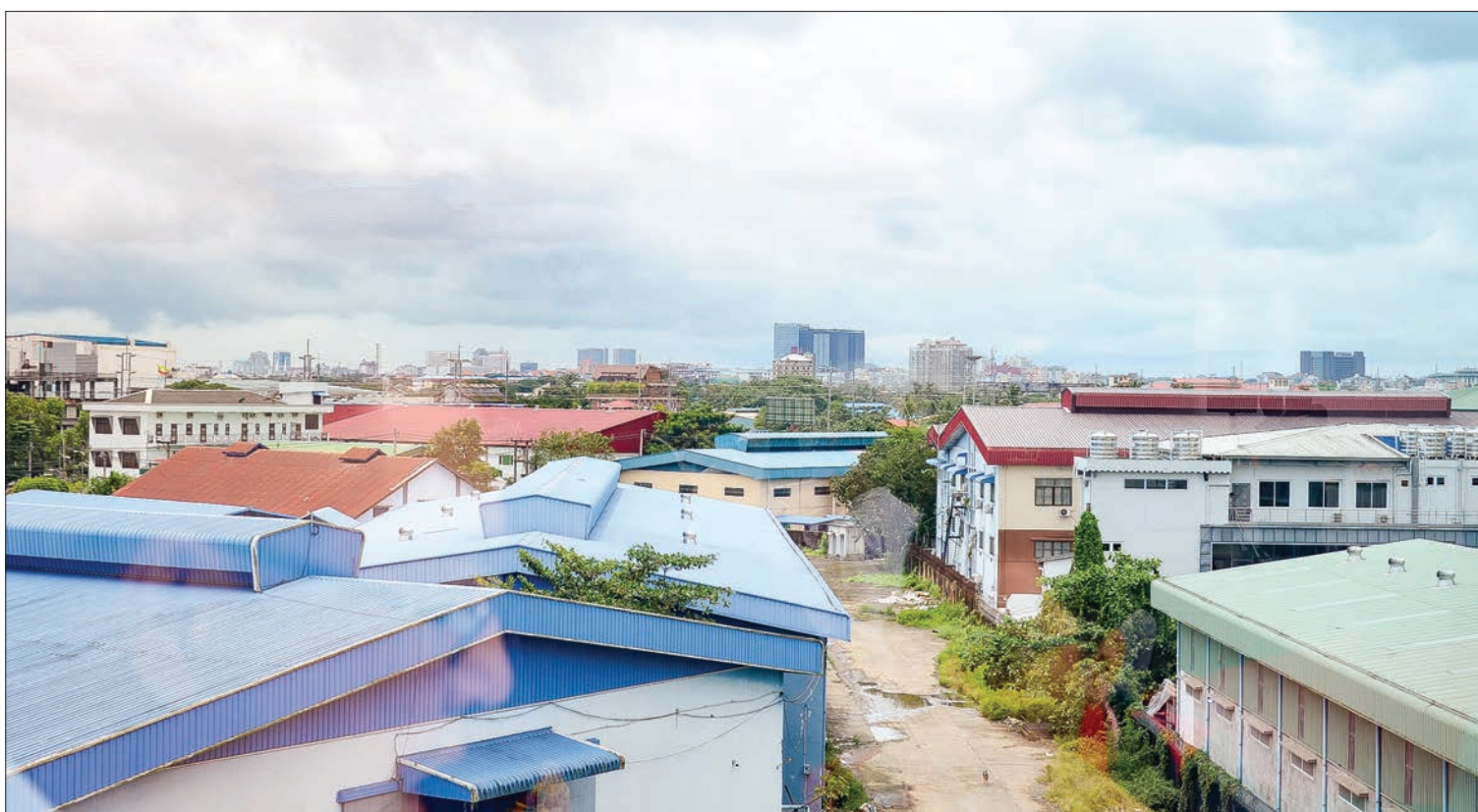
Buildings under construction at Tharkayta Industrial Park. PHOTO: PHOEKHWAR
