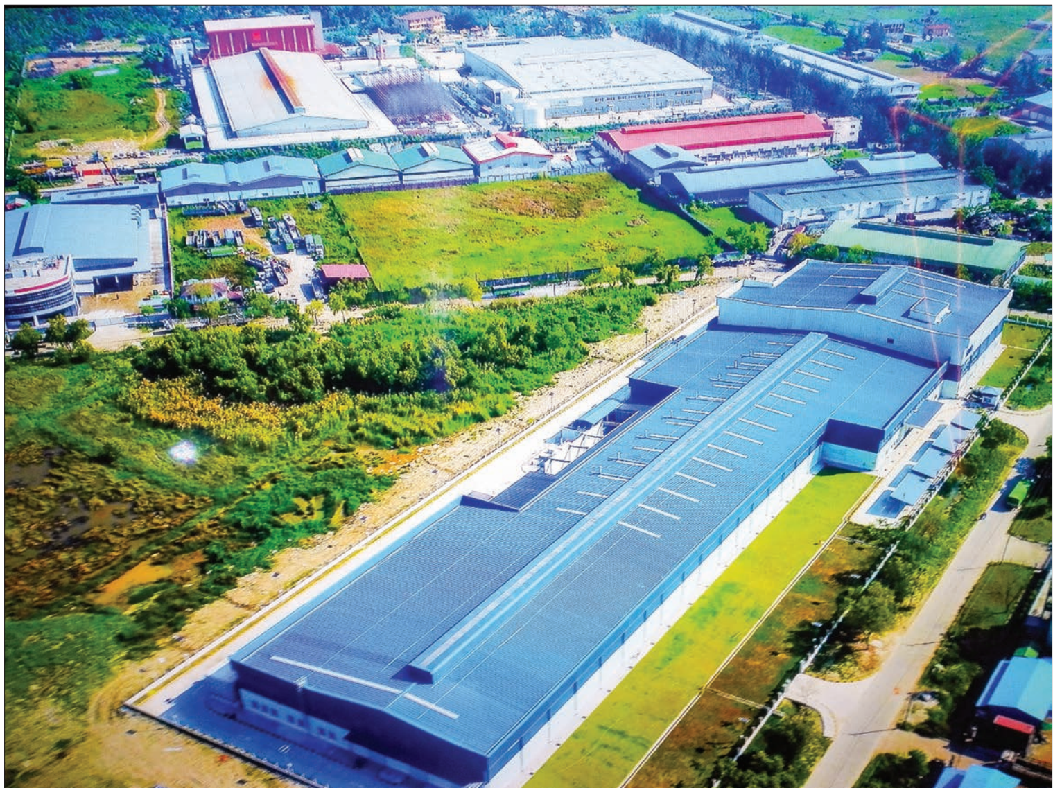
An aerial photo shows PEB Steel Myanmar's steel plant together with other industries in Thilawa Special Economic Zone. PHOTO: MYINT MAUNG SOE
