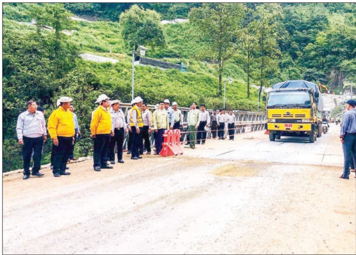
Officials witness the first traffic of 48-ton trucks over of the Gote Twin Bailey Bridge in Nawngkhio. PHOTO: KHAYAN SOE MYINT
