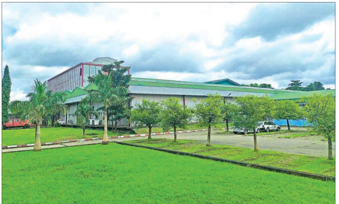
The building of Myanmar Pharmaceutical Factory in Insein Township, Yangon. PHOTO: MYINT
