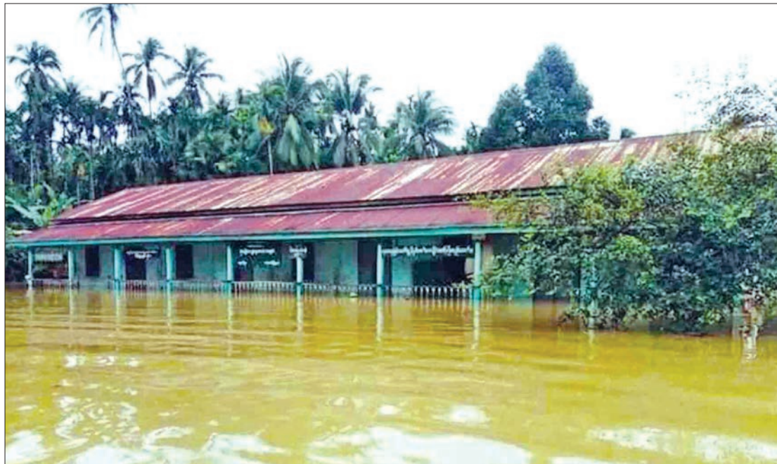
The school building is submerged by flood in Taninthayi Region. PHOTO: NAN THAR YE HTAIN WIN
