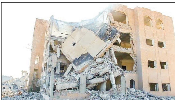
A screen grab from an AFPTV video shows the destroyed building following reported airstrikes on 1 September. PHOTO: AFP
