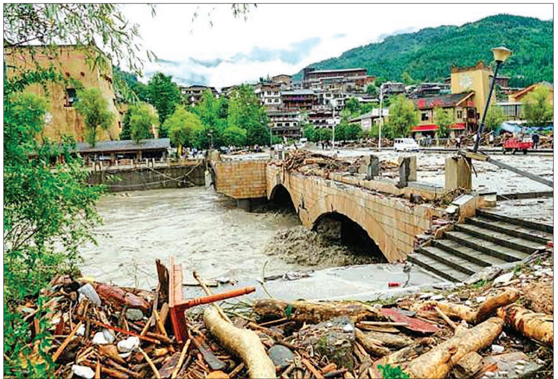
This photo taken on 21 August, 2019 shows the aftermath of a mudslide caused by heavy rainfall in Wenchuan county, in China's southwestern Sichuan province. PHOTO: AFP
