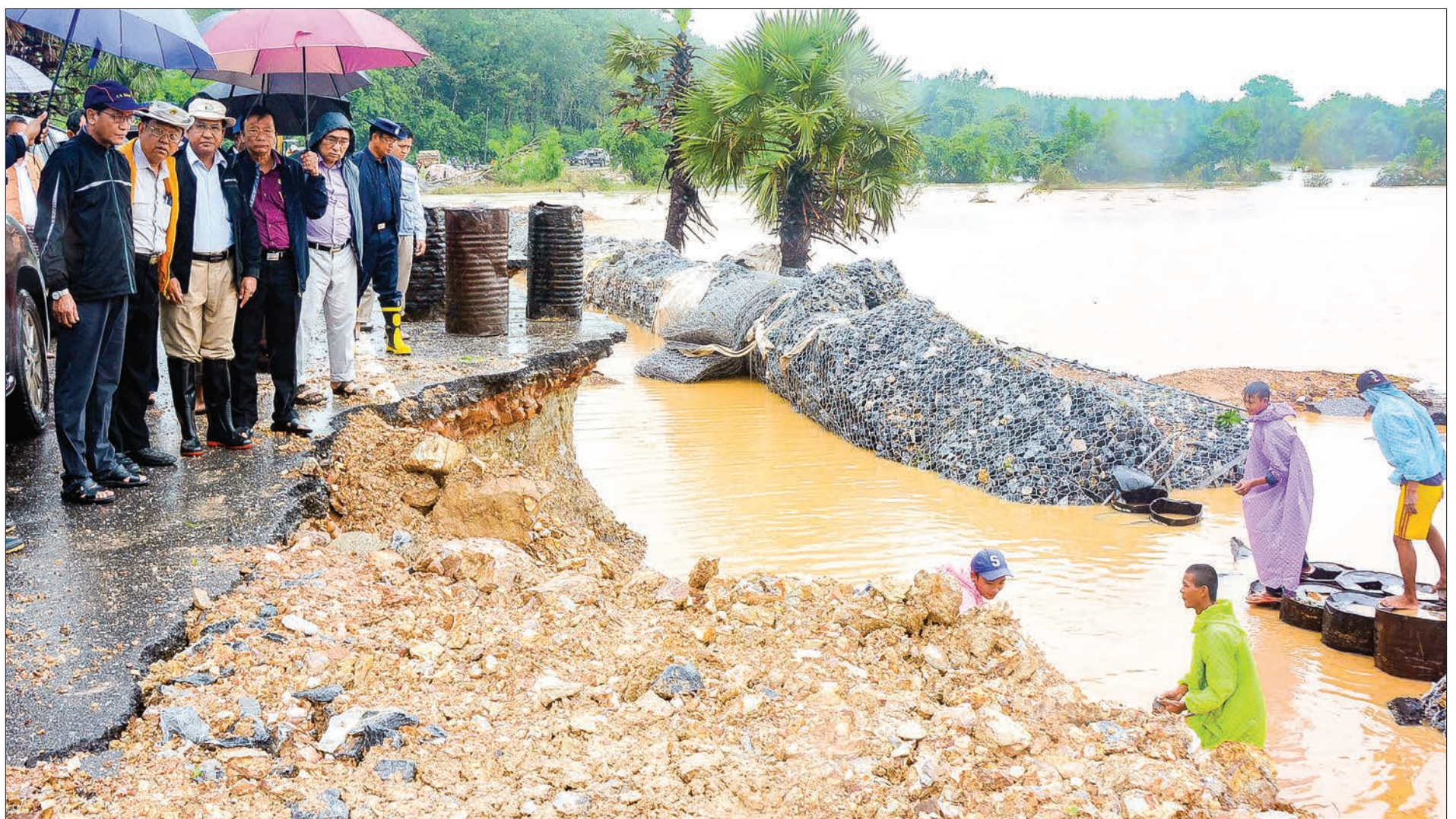
Vice President U Henry Van Thio inspects the damage of road section between Mile Post 45/46 and Mile Post 85 on Mawlamyine-Thanyuayay-ye Highway yesterday. PHOTO: MNA
