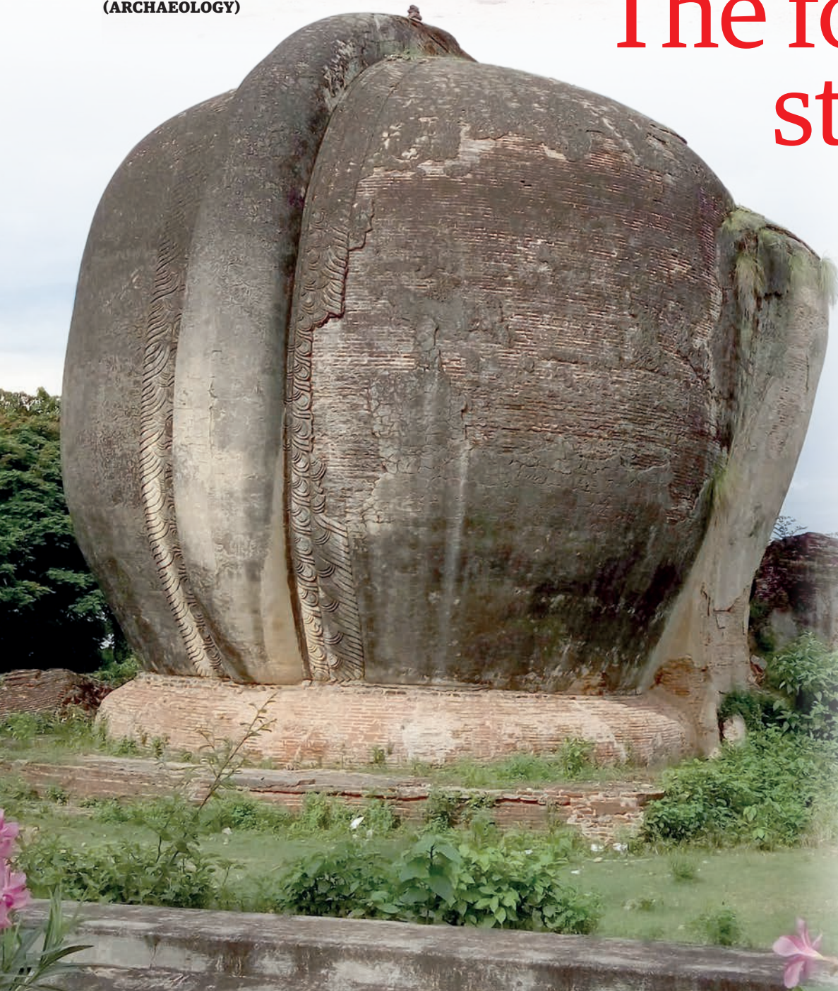
The Back part of the Gigantic Lion sculpture which destroyed by earthquake. PHOTO: MAUNG THA (ARCHAEOLOGY)
