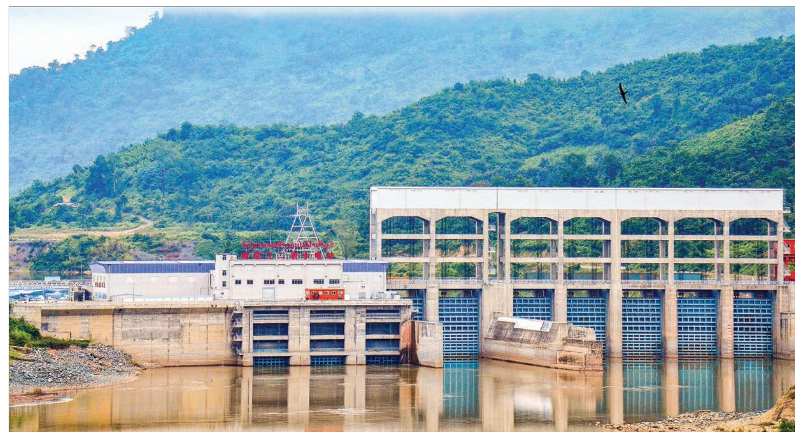
Photo taken on 12 Dec, 2016 shows the first stage's No. 2 hydropower station of the Power China-contracted project in Luang Prabang Province, north Laos. PHOTO: XINHUA
