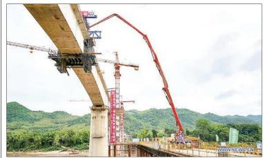
With the concrete beam of the last span over Mekong River put in place, the main section of Luang Prabang cross-Mekong River railway bridge has been completed on Sunday, seven months ahead of schedule. **PHOTO: XINHUA**
