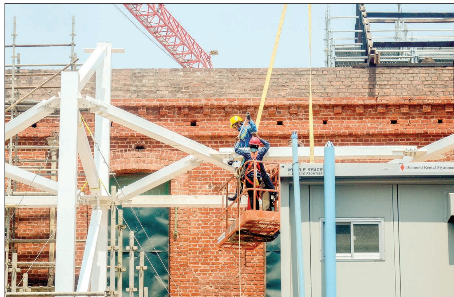
Workers at a construction site in Yangon. PHOTO: PHOE KHWAR
