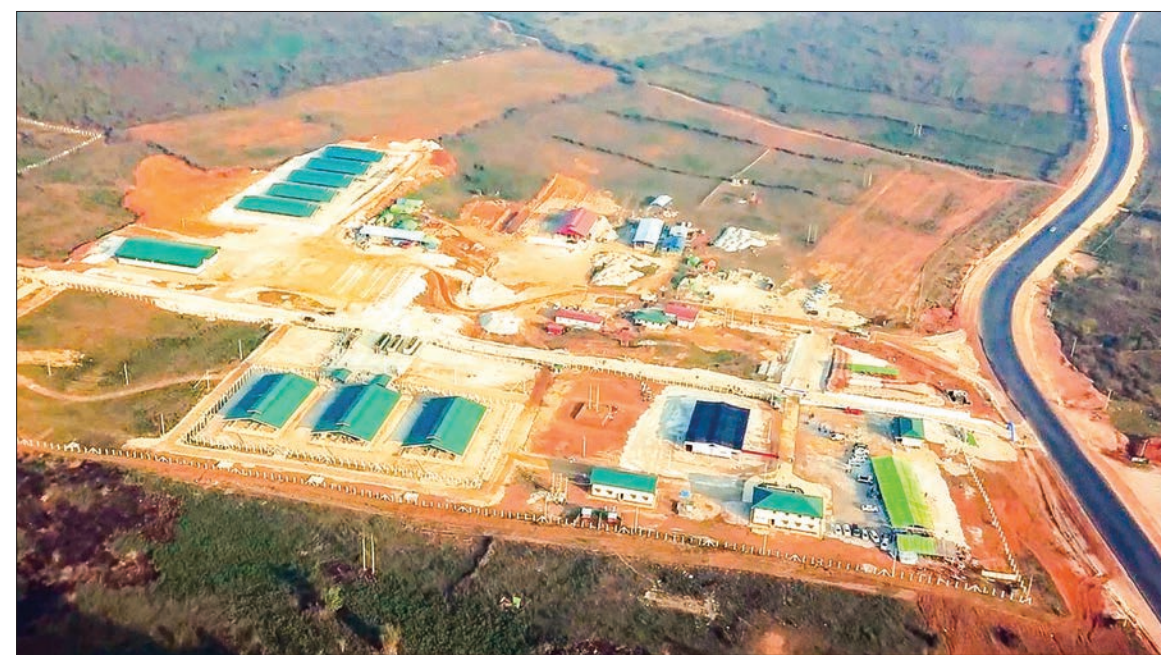
Buildings of the Animal Quarantine Station in Kutkai.
