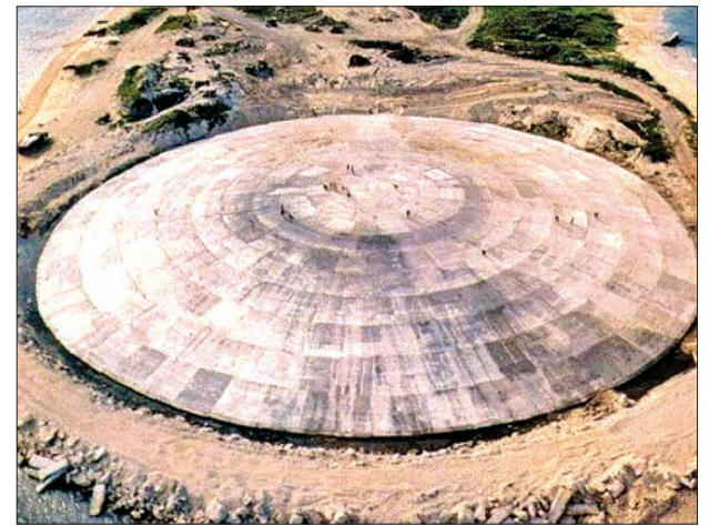
A huge concrete dome built over a crater left by one of the 43 nuclear blasts on Runit Island photographed in 1980. PHOTO:AFP
