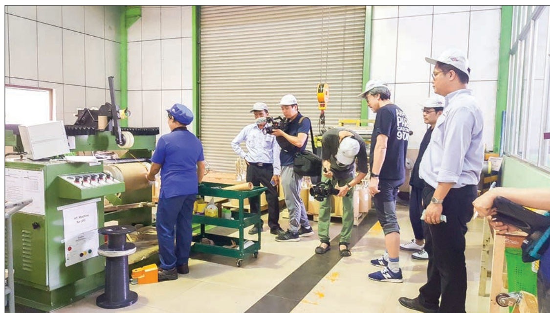
Japanese film crew shoots production of transformer at a factory in South Dagon Industry Zone in Yangon yesterday. PHOTO: MNA
