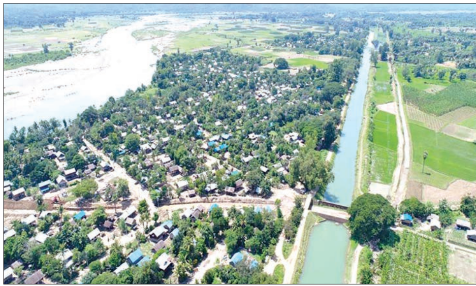
Ingone canal in Ingone Village, Pwintbyu Township under construction.
