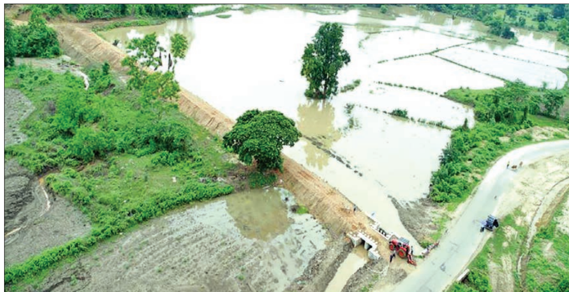
Tawmon lake near Tawmon Village, Thayet Township under renovation.
