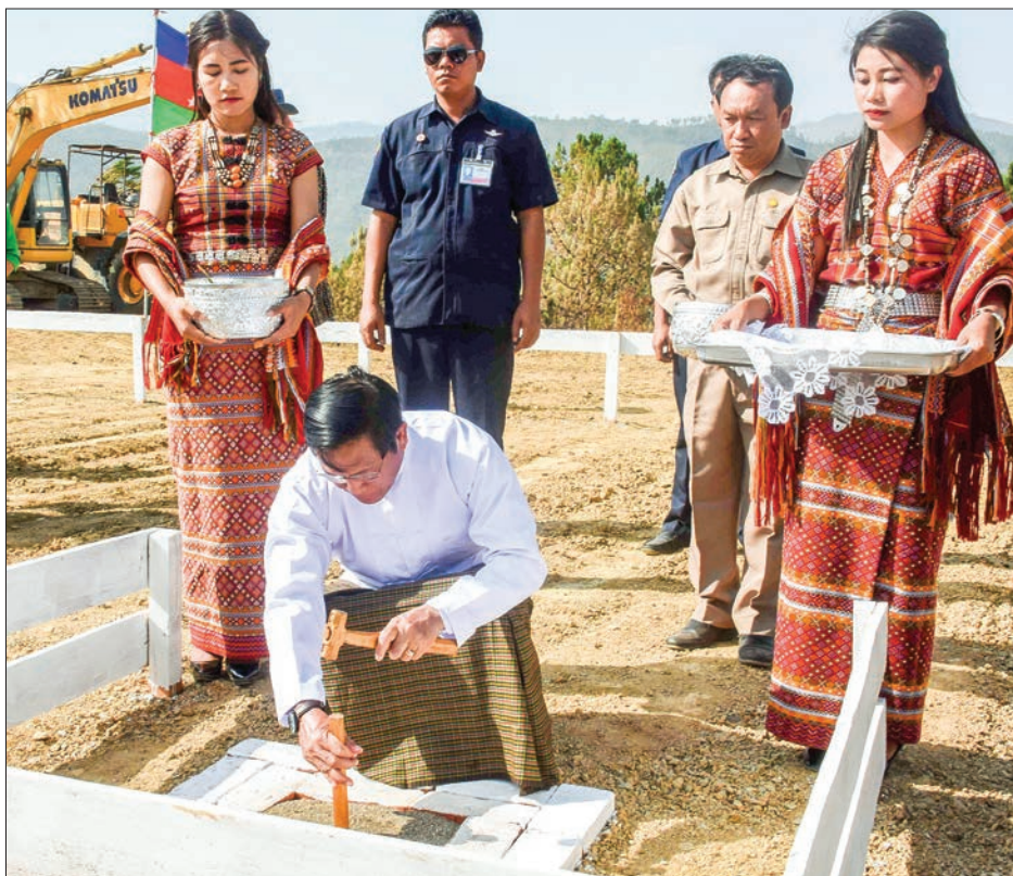
Vice President U Henry Van Thio drives a stake at the construction location for the administration office of the Sports and Physical Education Institute (Haka). PHOTO: MNA
