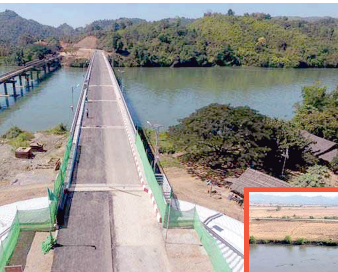
Darlet Creek Bridge. PHOTO: TIN TUN (IPRD)
