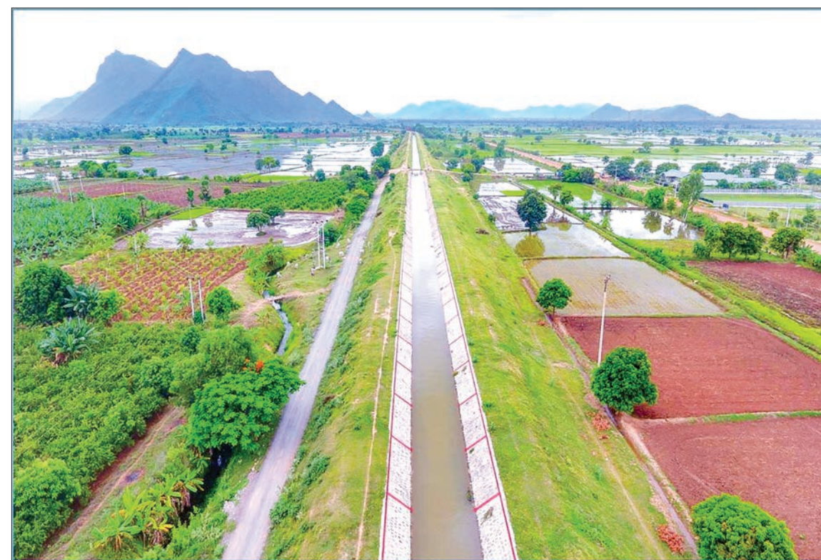
Shwe Hlan Bo River Pumping Station irrigates the farmlands Singaing Township.
