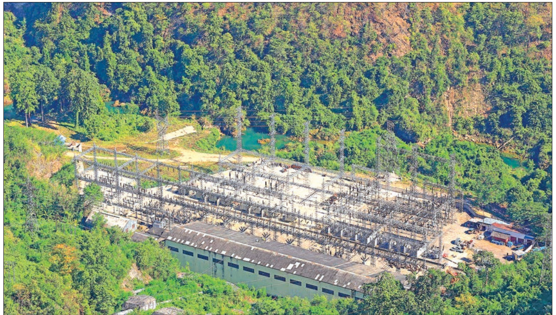
Balu Chaung Hydropower Station No. 2
