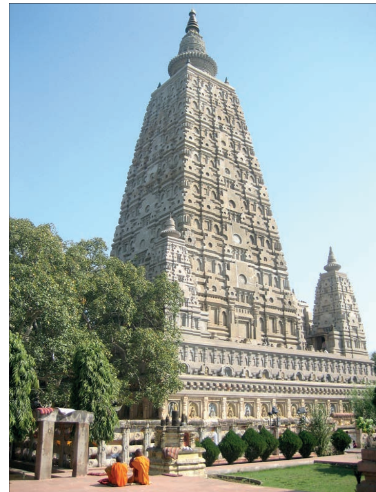
Mahabodhi temple, built under the Gupta Empire, 6th century CE.
