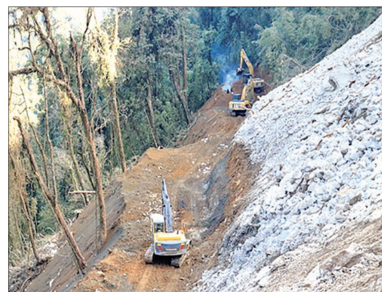
Machines paving into the Maggwayza-Khaunglanphu road section.
