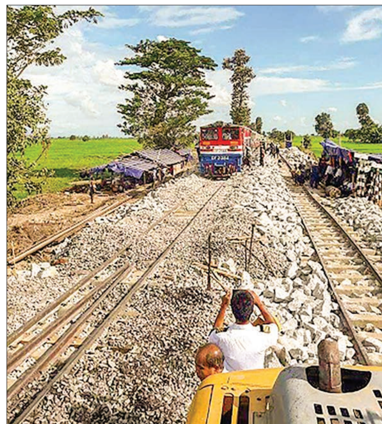
Rail workers are upgrading the rail tracks around the country.
