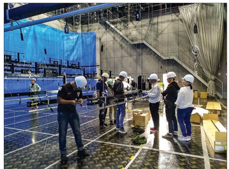
Workers install broadcasting equipment at the MRTV.
