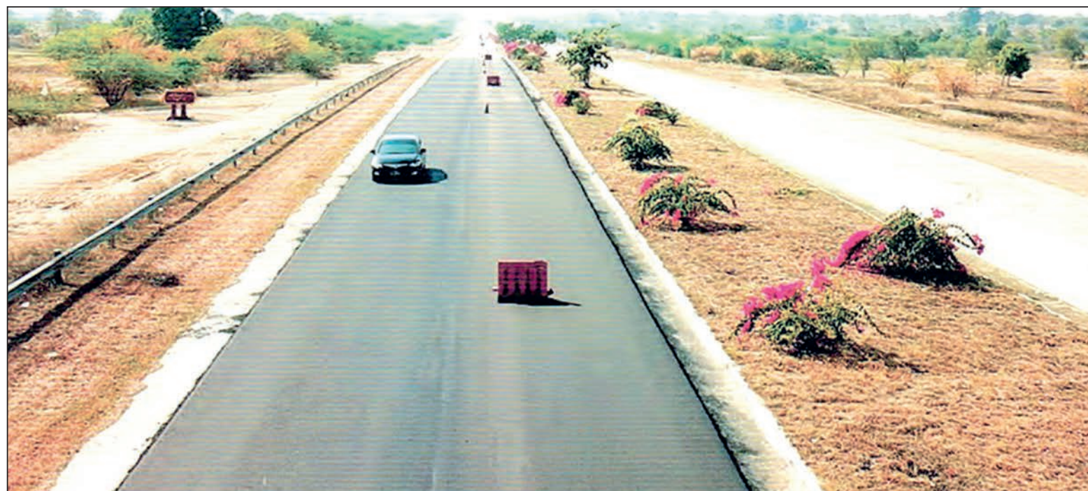
The Yangon-Mandalay highway is upgraded as asphalt road.
