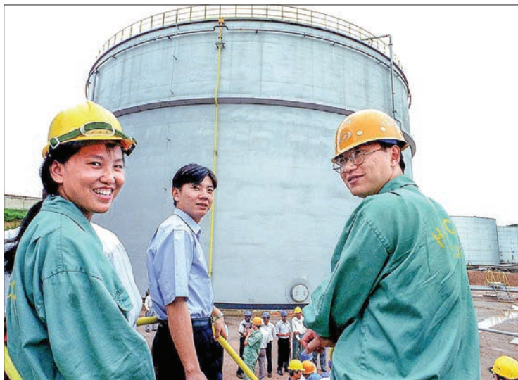
File photo shows workers stand in front of a new oil storage tank in Sri Lanka. PHOTO: AFP
