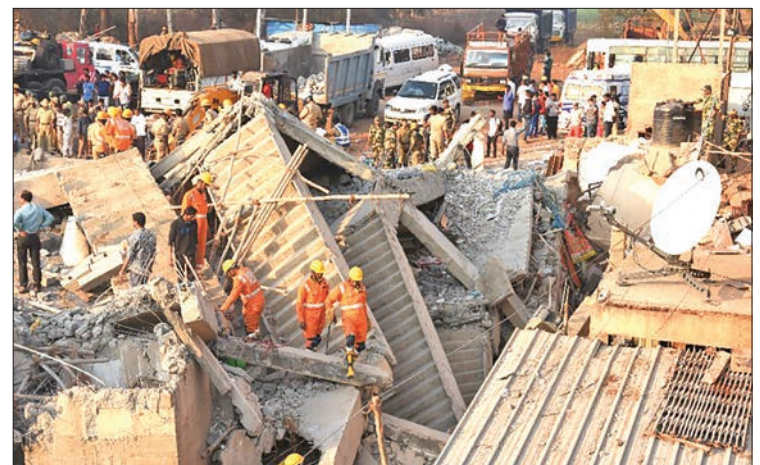
Around 400 rescuers have been scouring through tonnes of concrete and steel after the building collapse. PHOTO: AFP
