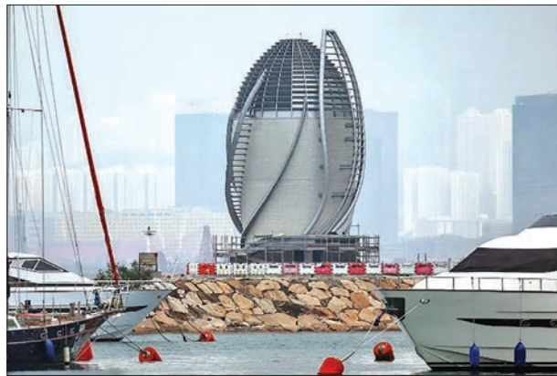
This this photo taken on March 17, 2019, the leaf-shaped ventilation shaft (C) for the air purification system of the Central-Wan Chai bypass tunnel is seen beyond anchored boats in Hong Kong. HOTO: VIVEK PRAKASH / AFP
