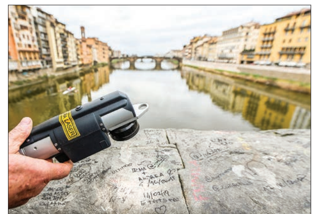
A volunteer from the Beauty Angels (Angeli del Bello) environmental association, a group that aims at keeping the Tuscan capital clean of graffiti, uses a powerful laser blaster to remove graffiti from the Ponte Vecchio medieval arch bridge over the Arno river on 7 March 2019 in Florence, Tuscany. PHOTO: AFP
