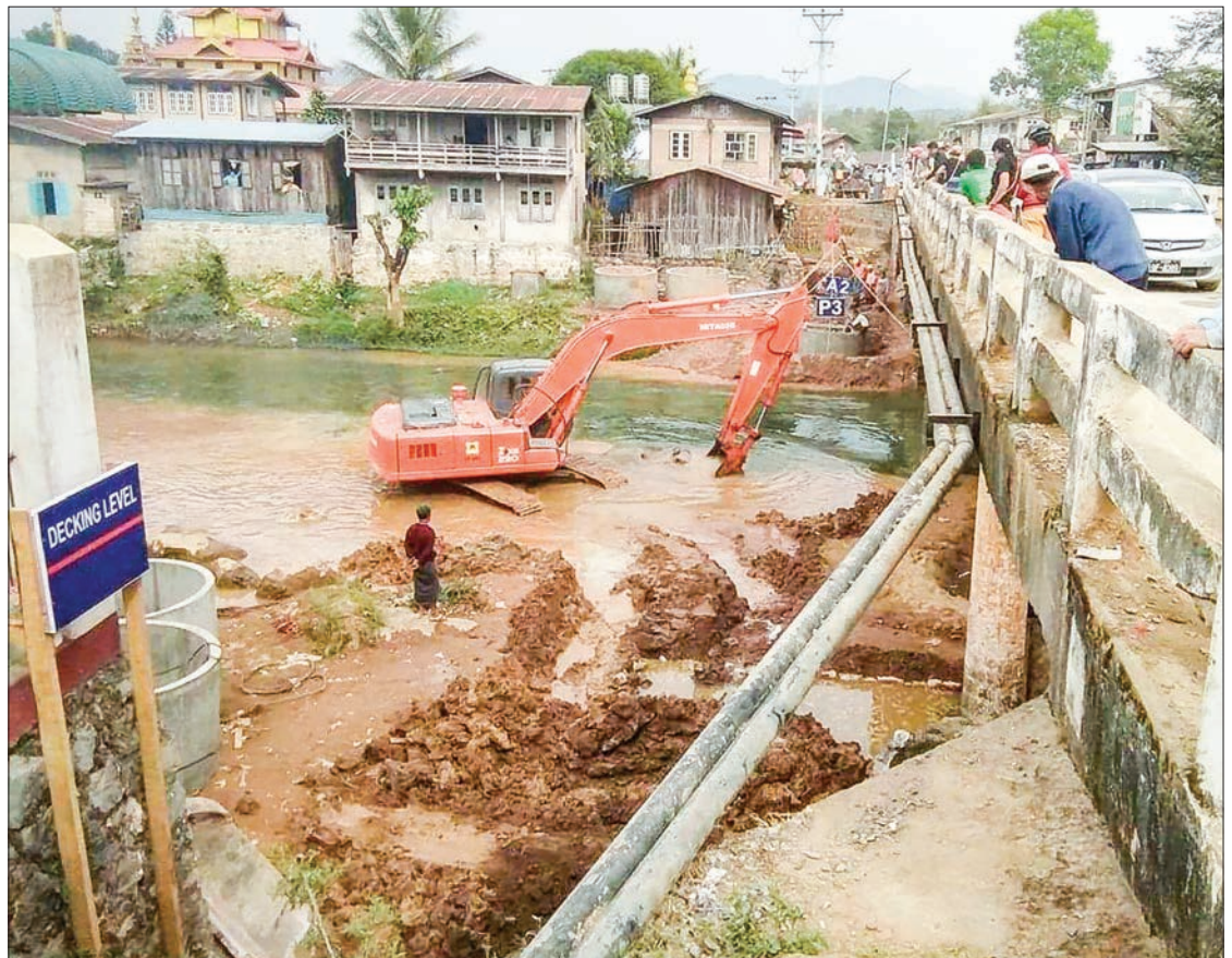
Construction work underway at the reinforced concrete bridge in Mongshu Township.
