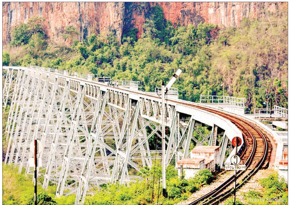
A new four-lane section of the Mandalay-Lashio-Muse motor road will be constructed, along with a bridge near the Goteik Viaduct. PHOTO: SUNSHINE
