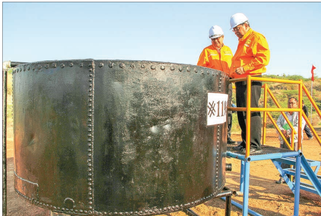
Union Minister U Win Khaing (Right) inspects a oil tank as he visits Chauk oilfield in Magway. PHOTO: MNA
