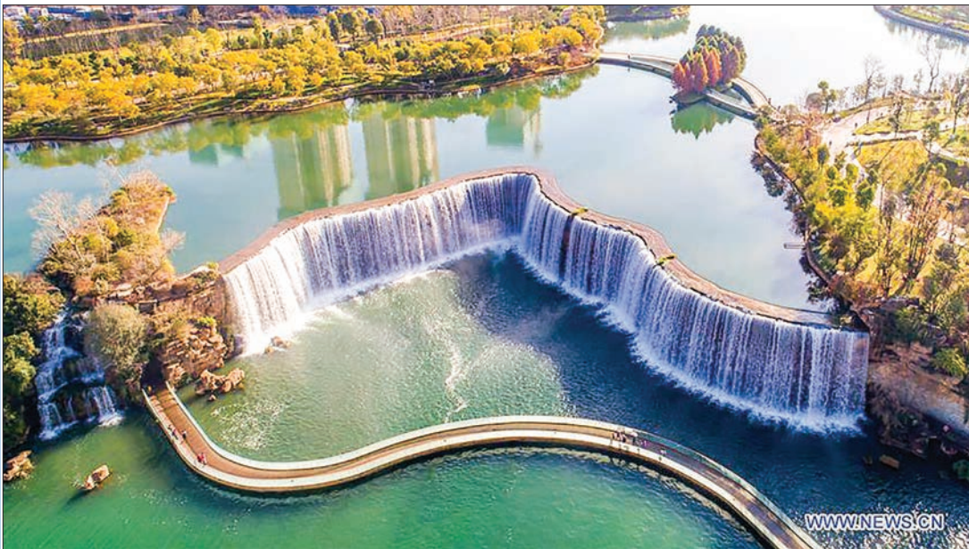
Aerial photo taken on 5 January, 2019 shows scenery of Kunming Waterfall Park in Kunming, capital of southwest China's Yunnan Province. The park features a grand manmade waterfall, which is 12.5 metres in height and 400 metres in width. The waterfall is part of the project diverting water from the Niulan River into Dianchi Lake. PHOTO: XINHUA
