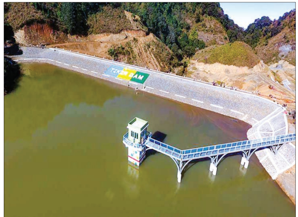
Tikir Dam near Thantlang Town and Tikir Village in Chin State is 500-foot-long and 75-foot-high and can store 1,265 acre feet of water to 12 villages and produces 50 kilowatts of electricity through a mini-hydroelectric power station. PHOTO: MNA
