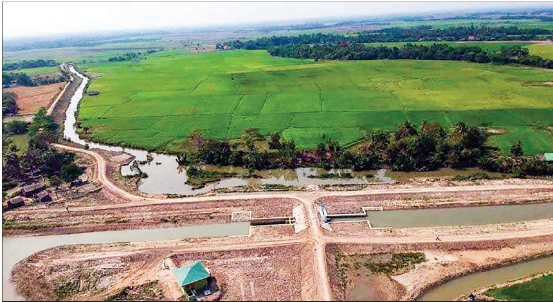
The sluiceways built between the Yway and Pyamalok Rivers will filter out seawater for monsoon and summer paddy cultivation in the Ayeyarwady Region. PHOTO: MNA
