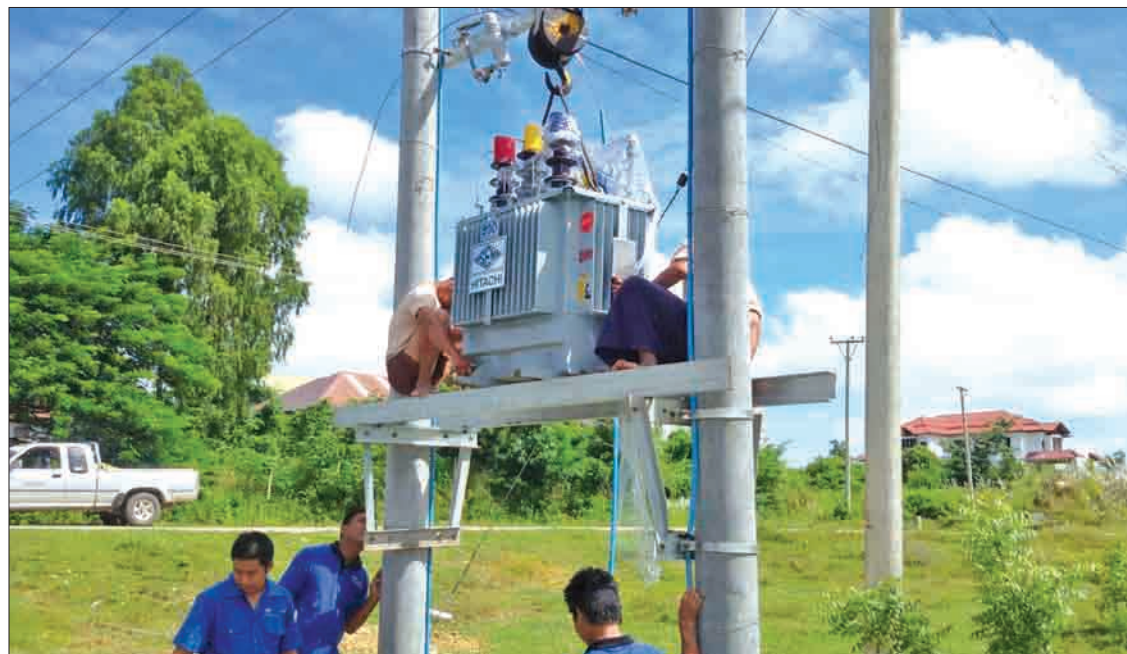
Workers assemble a 200 KVA transformer for the Sub-power station-1 in Dakkhinathiri Township in Nay Pyi Taw Council Area. FILE PHOTO
