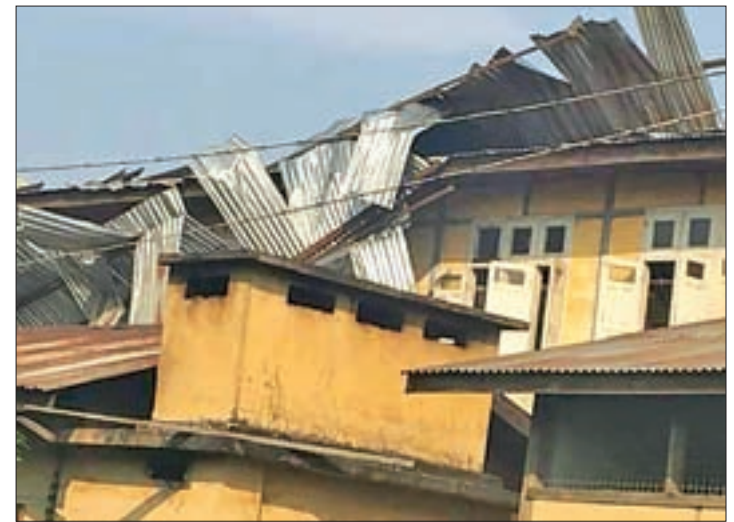
The house damaged by the strong wind in Hakha . PHOTO: KYAW SWAR FB
