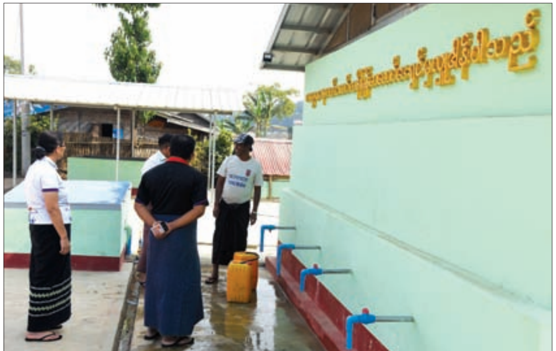
Kanbawza's drinking water supply facility being seen in Aungban. PHOTO: GNLM
