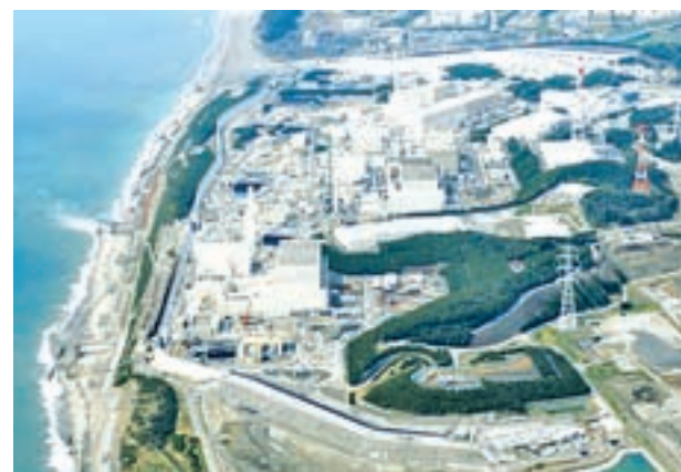
Chubu Electric Power Co's Hamaoka nuclear plant in central Japan: Construction of a coastal levee to protect against tsunami from a possible Nankai Trough earthquake will be completed on 31 March. PHOTO: KYODO NEWS
