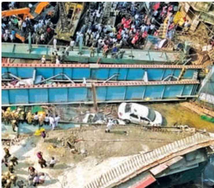
A general view of the collapsed flyover in Kolkata, India, on 31 March. PHOTO: REUTERS
