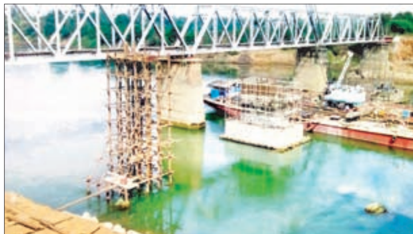
Photo shows Myitnge Rail Bridge which is under construction. PHOTO: TIN MAUNG LWIN (MYANMA ALINN)
