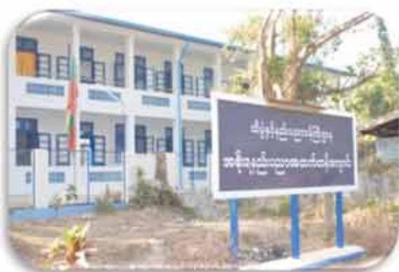
Upgraded Government Technical High School in Dawei
